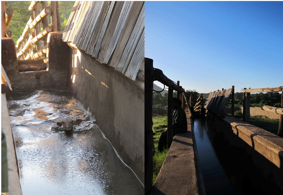
Figure 6. Makushane dip tank. In the image the path leading to the tank can be seen, as well as a young cattle swimming in the veterinary mix.
