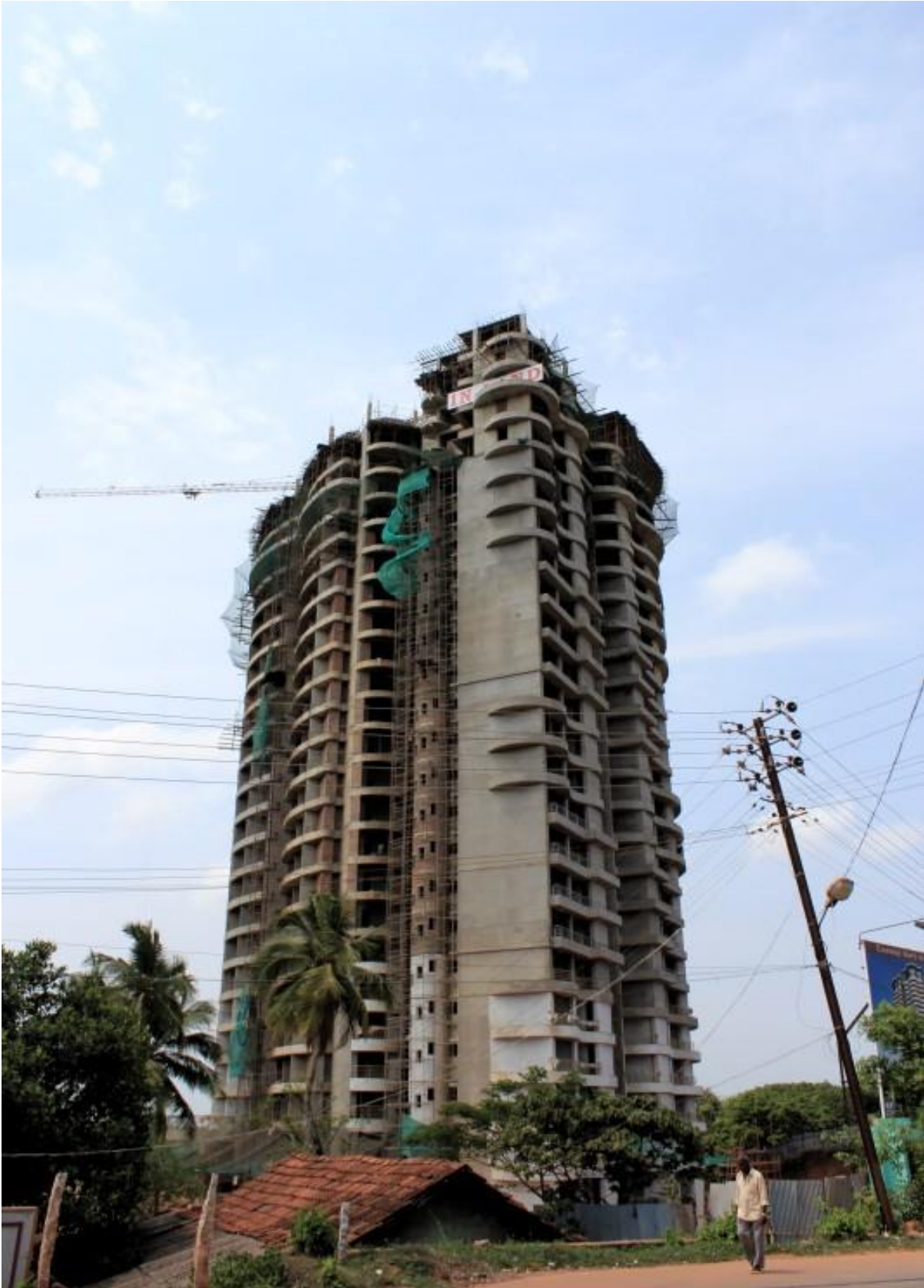
Figure 15: A building under construction. Source: Author.
