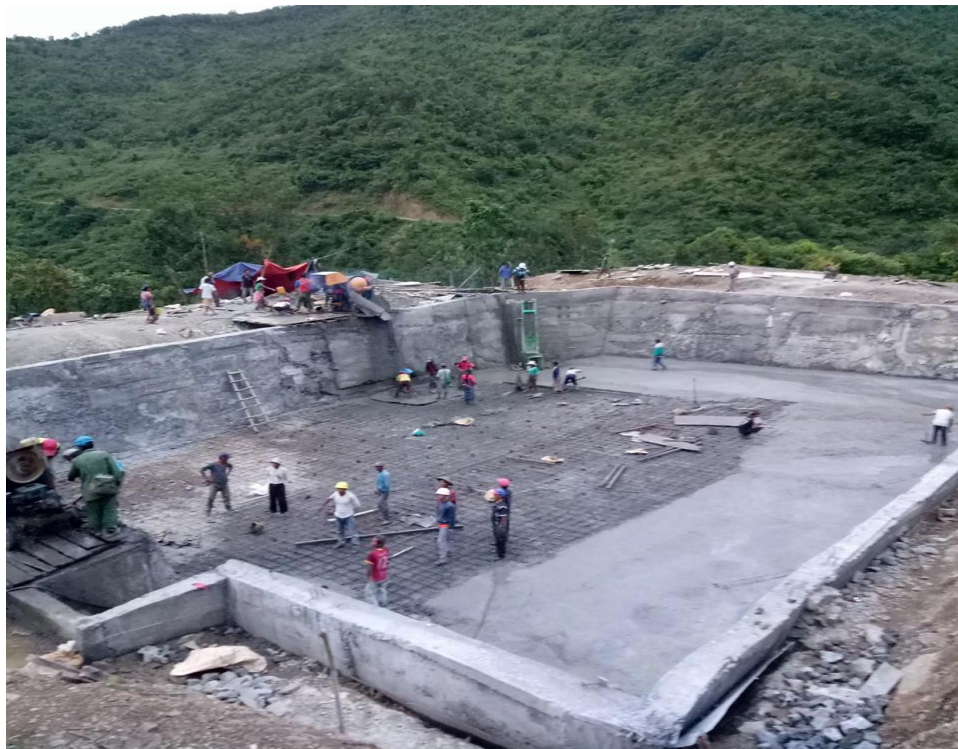
Figure 5: Water storage construction for micro-hydropower plant in Aibur village
