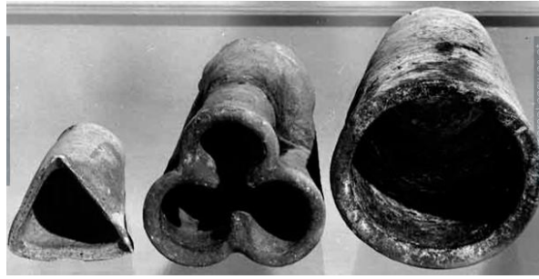
Fig.1.13. Bowl-shaped tiles with triangular, three-lobed and circular openings. 45
