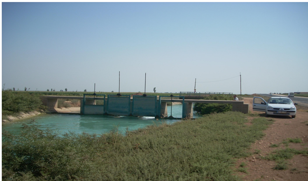
Figure 6.3 Main irrigation channel with water gates for irrigation of fields, Harran, GAP
