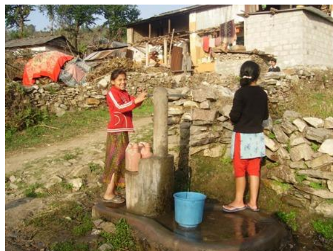
Tapstands for domestic water usage
