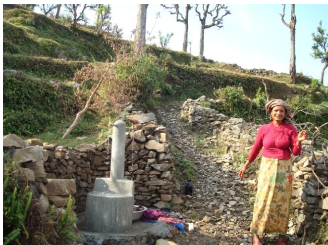
Tapstands for domestic water usage
