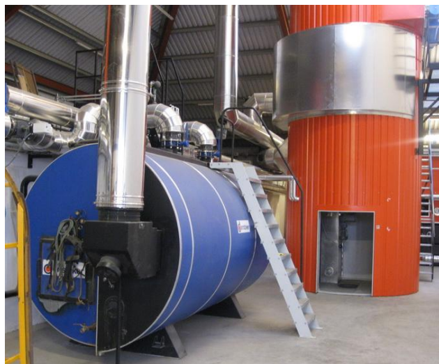
Figure 5-10. Flue gas cleaning and reserve oil boiler at Stokkemærke neighbour heating plant, Denmark
