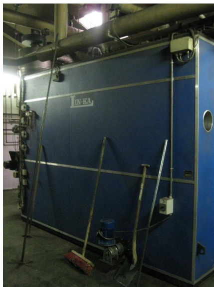
Figure VI-3. 1 MW straw-fired boiler on Horreby farm, Denmark
