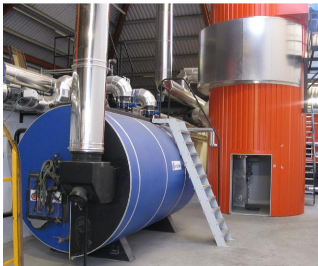
Figure VI-11. Flue gas cleaning and reserve oil boiler at Stokkemærke neighbour heating plant, Denmark
