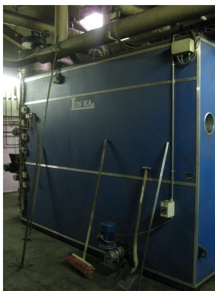
Figure 5-2. 1 MW straw-fired boiler on Horreby farm, Denmark
