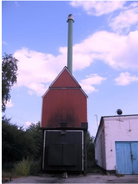
Figure 2-3. Batch-fired straw boiler with hot water accumulator
