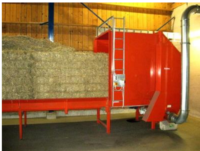
Figure VI-2. A straw conveyor and shredder supplying fuel to the boiler at Svenstorp estate, Scania, Sweden
