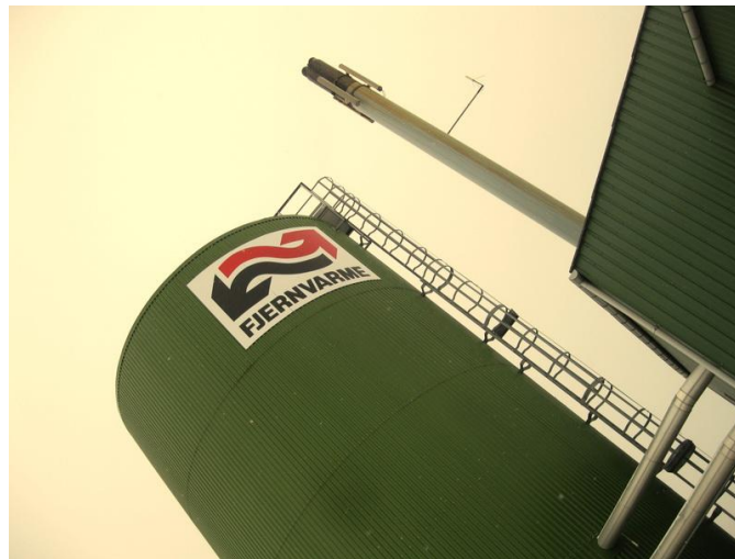
Figure VI-6. 550 m 3 hot water accumulator at Horbelev neighbour heating plant, Denmark
