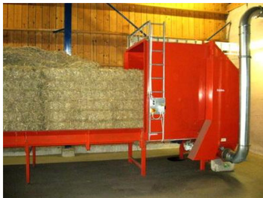
Figure 5-3. A straw conveyor and shredder supplying fuel to the boiler at Svenstorp estate, Scania, Sweden
