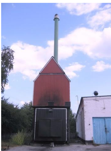
Figure VII-4. 980 kW straw-fired boiler RAU-2-1210 in Drozdy village, Kyiv province, Ukraine
