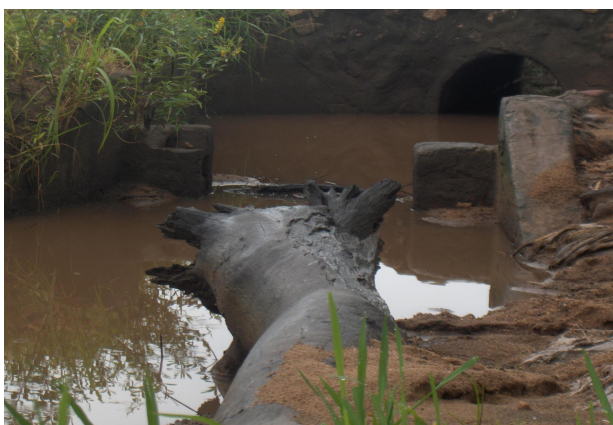
Figure 7.11: A wood log and sand in a secondary canal
