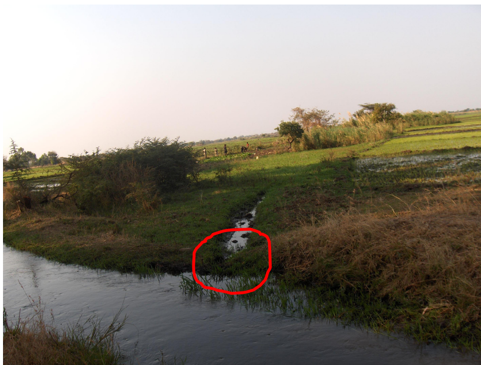
Figure 5.15: An illegal access point on a secondary canal
