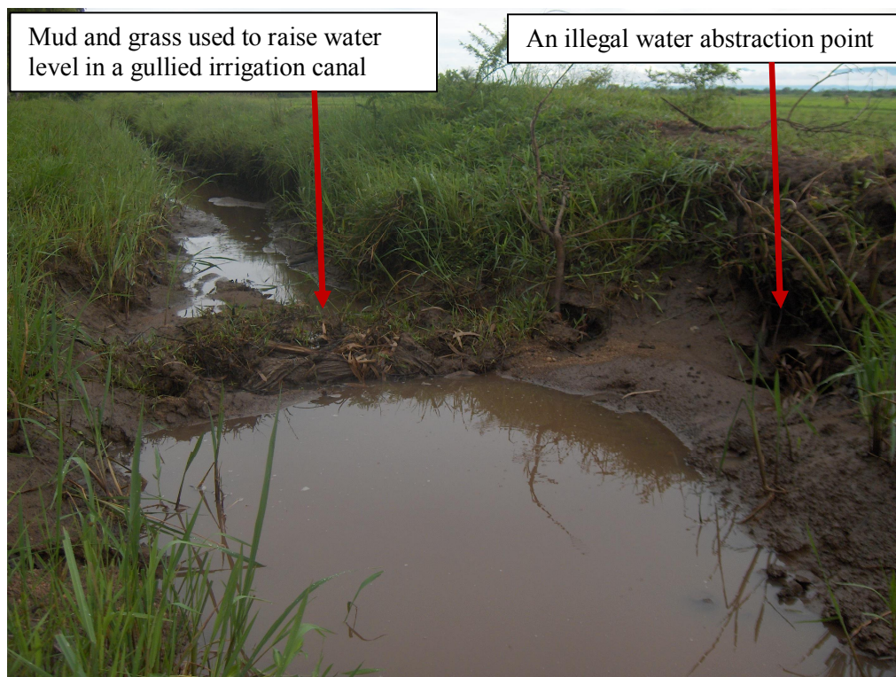
Figure 8.2: A canal in Wovwe I turned into a gully
