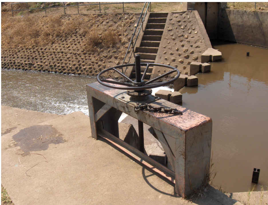
Figure 5.12: Unlocked water gate at the Headworks intake
