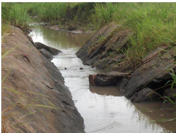
Figure 7.13: Broken concrete on a segment of a weedy main canal from headworks
