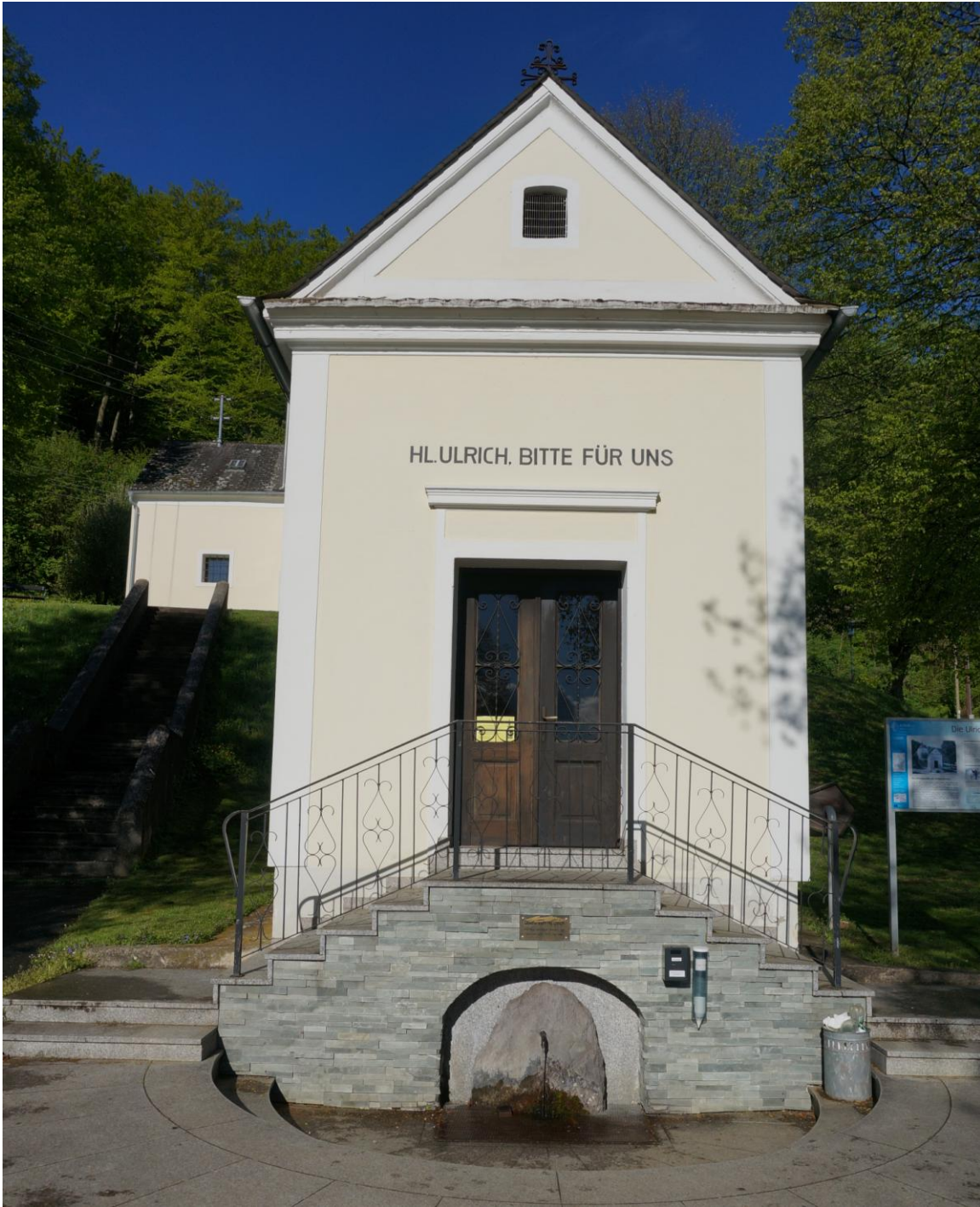
Figure 16. St. Ulrich's Well and Chapel. Clement's Church can be seen behind.
