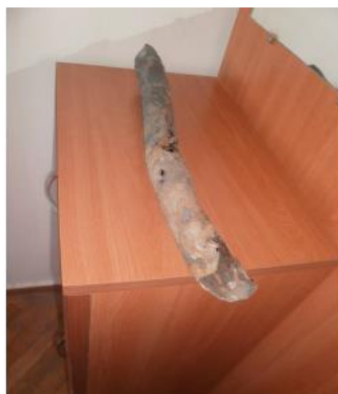
Picture 5. Water pipe changed during repair: Photo by Naira Harutyunyan
