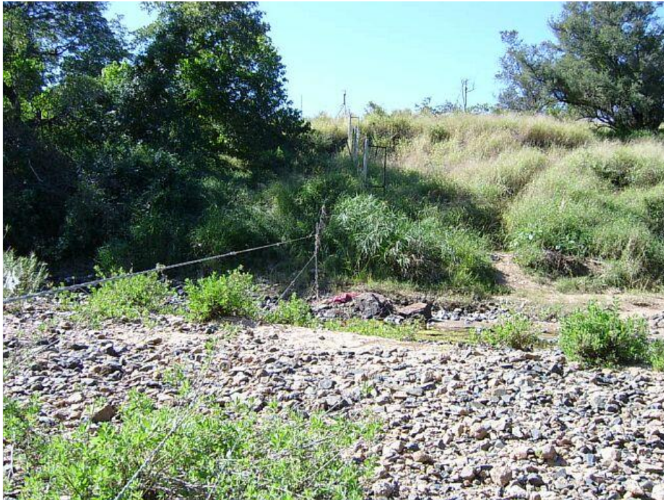
Figure 7.24: Inadequate KNP border fencing across Shingwedzi River, consisting of a mere three strands of barbed wire.
