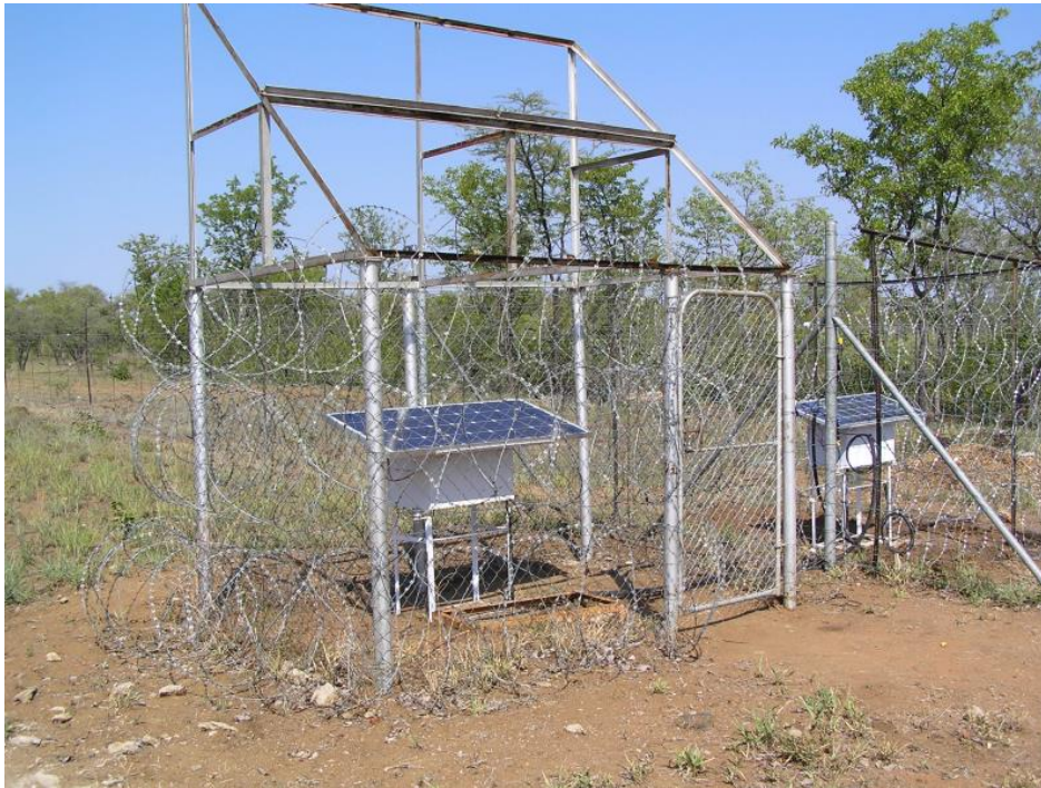
Figure 7.23: New solar panels to provide electrification for KNP border fence, protected by barbed wire, were needed to replace stolen panels (empty frames at top of structure).
