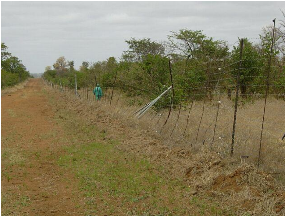
Figure 7.22: Fence maintenance is hindered by limited access due to dense vegetation.
