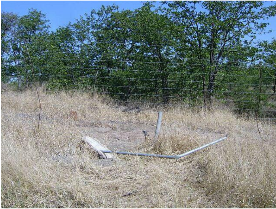
Figure 7.18: Elephant are able to push and/or pull down KNP border fence poles which, due to their hollow design, easily bend or crack.
