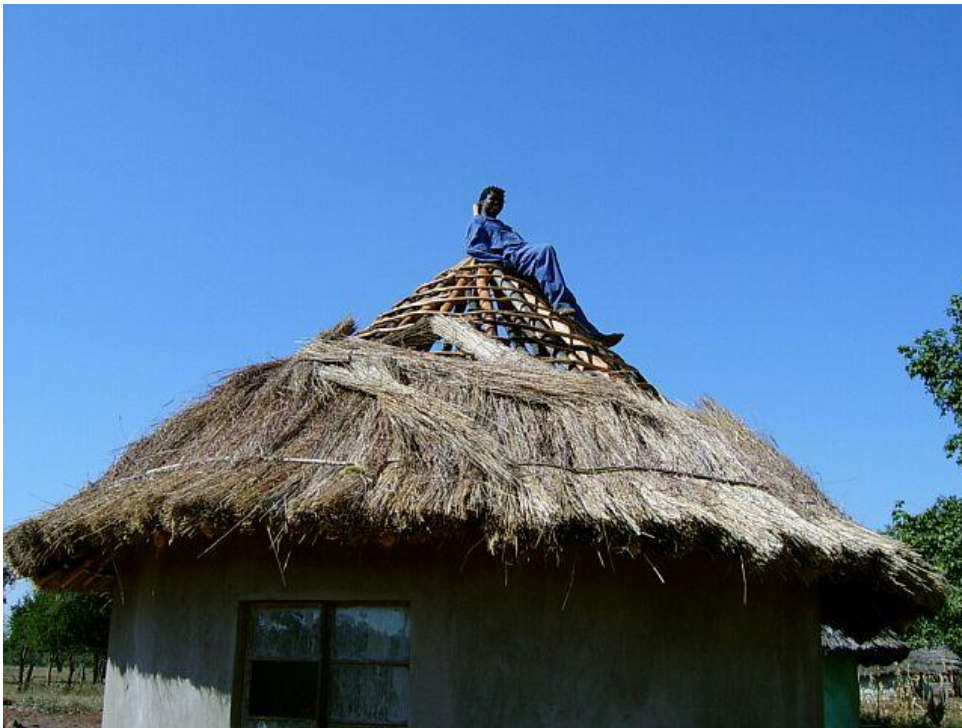
Figure 4.16: Traditional Tsonga hut being constructed in Mahlathi village. Roofs are assembled from timber poles and ‘bundles’ of thatch grass.
