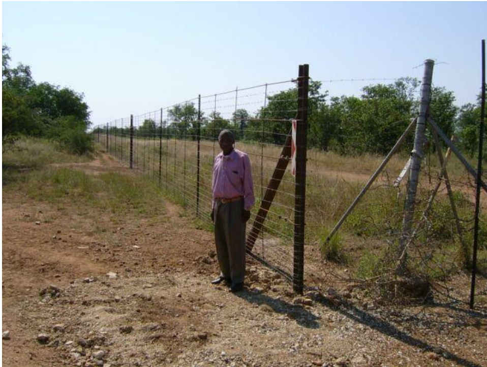
Figure 7.25: New 'human-friendly' KNP border fence constructed north of Lombaard village.
