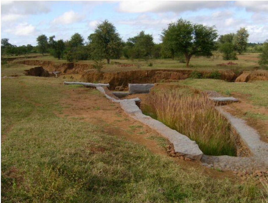
Figure 6.8: Streambank stabilization project near Matiyani village
