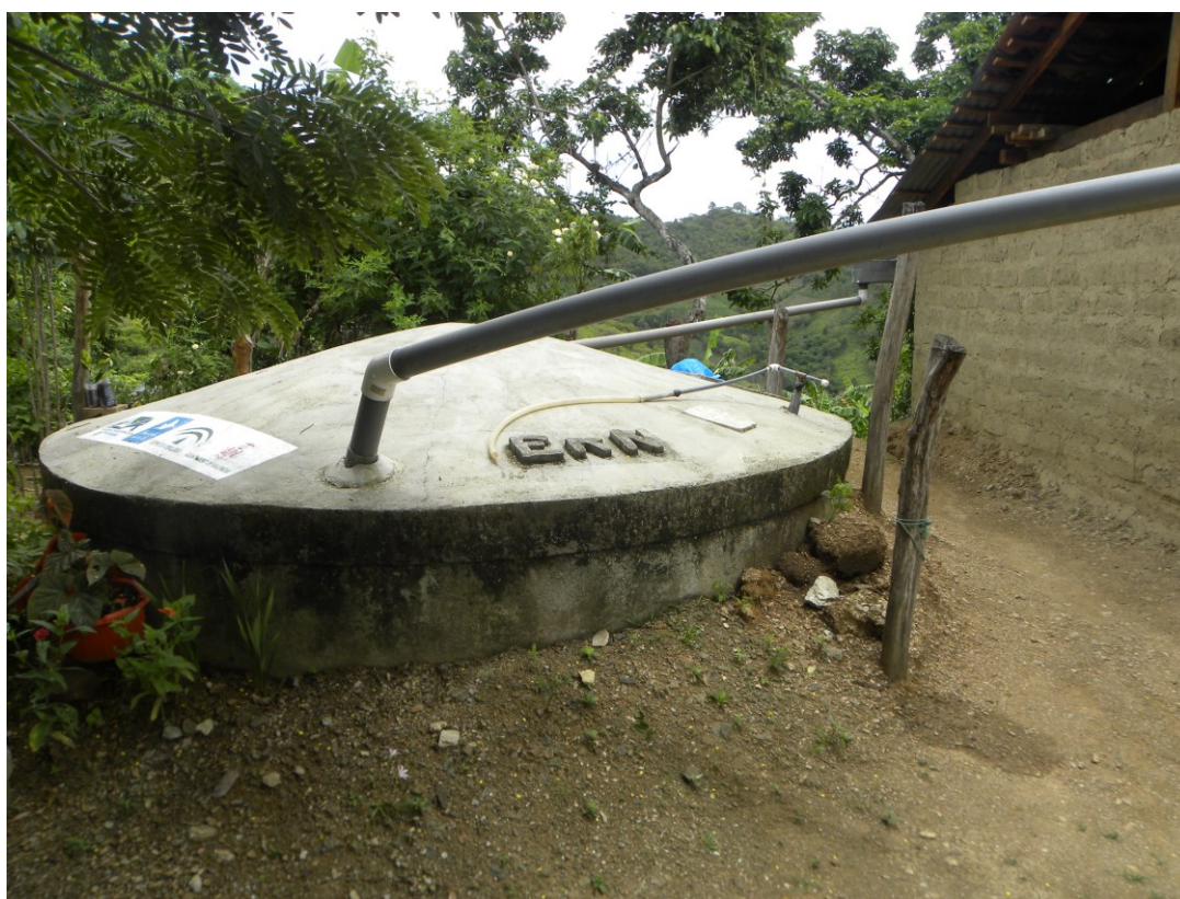
Picture 21. Water reservoir for rainwater harvesting in El Nancite
