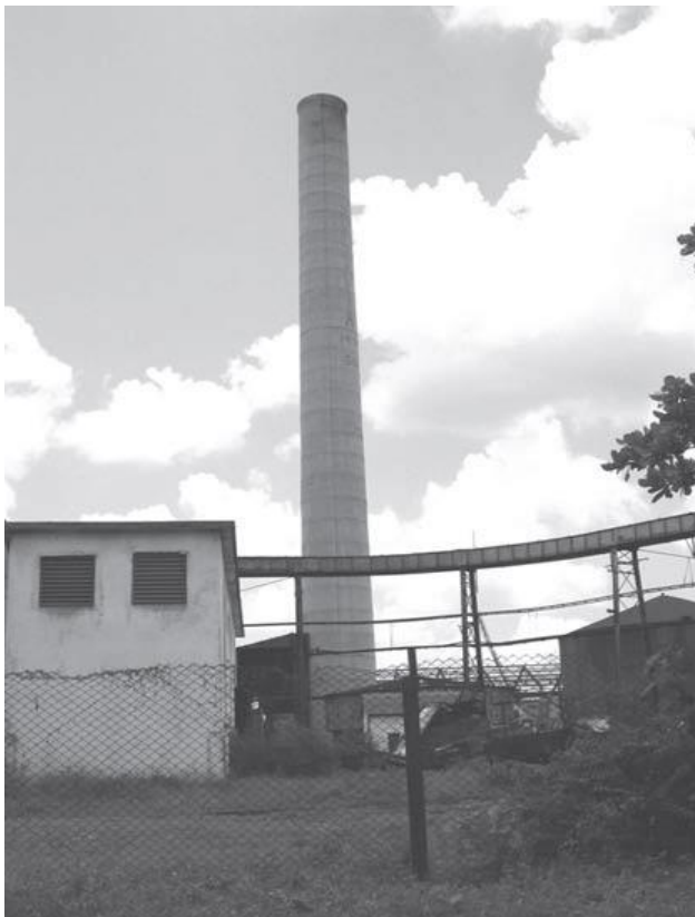
Figure 11. A Closed sugar mill in Ciego de Avila. It shows the chimney and elevated cane-loading belt. Source Scarpaci & Portela 2009
