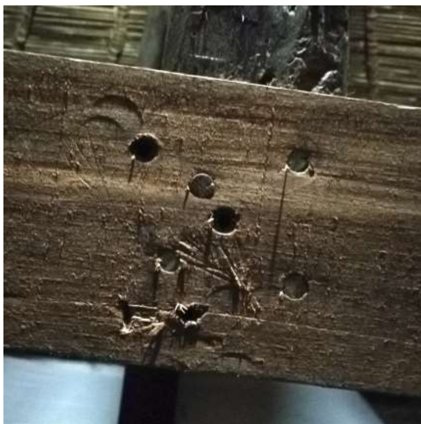
Figure 14. Nails I found in one of the Dukligan hut’s beams. Photo taken by the author.
