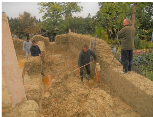
Figure 32: Building cob walls: working in pairs Source: Gáspár János, “Képgaléria - újra itt a vályogfal ideje! [Gallery- The Time of Earth Walls Is Here Again!],” accessed 5 May 2019, https://valyogfal.hu/kepgaleria/ .
