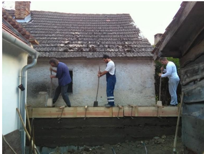
Figure 36: Ramming earth wall in Nagyvázsony Source: Photo made by Ádám Bihari, in Nagyvázsony, 2018
