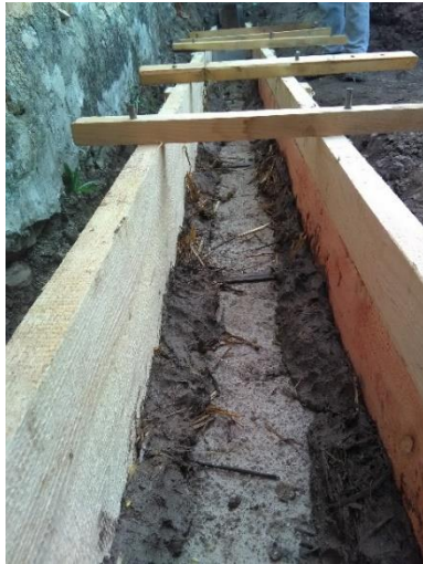
Figure 35: Shutters on rammed earth wall, straw-earth placed on the edges Source: Photo made by Ádám Bihari, in Nagyvázsony, 2018
