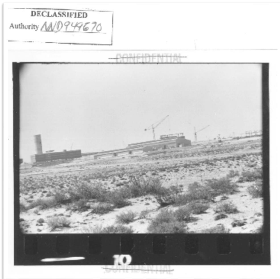
Figure 3.2 Dimona construction site in late 1960
