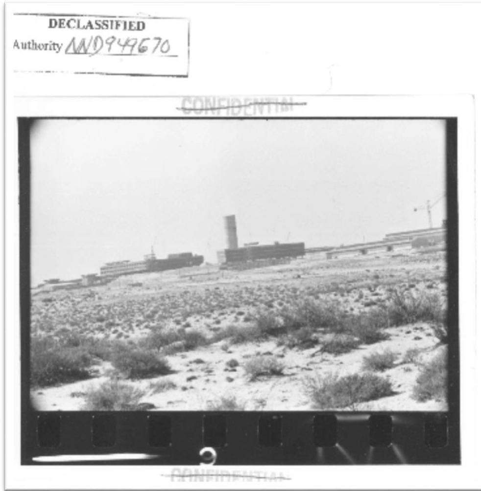
Figure 3.3 Dimona construction site in late 1960
