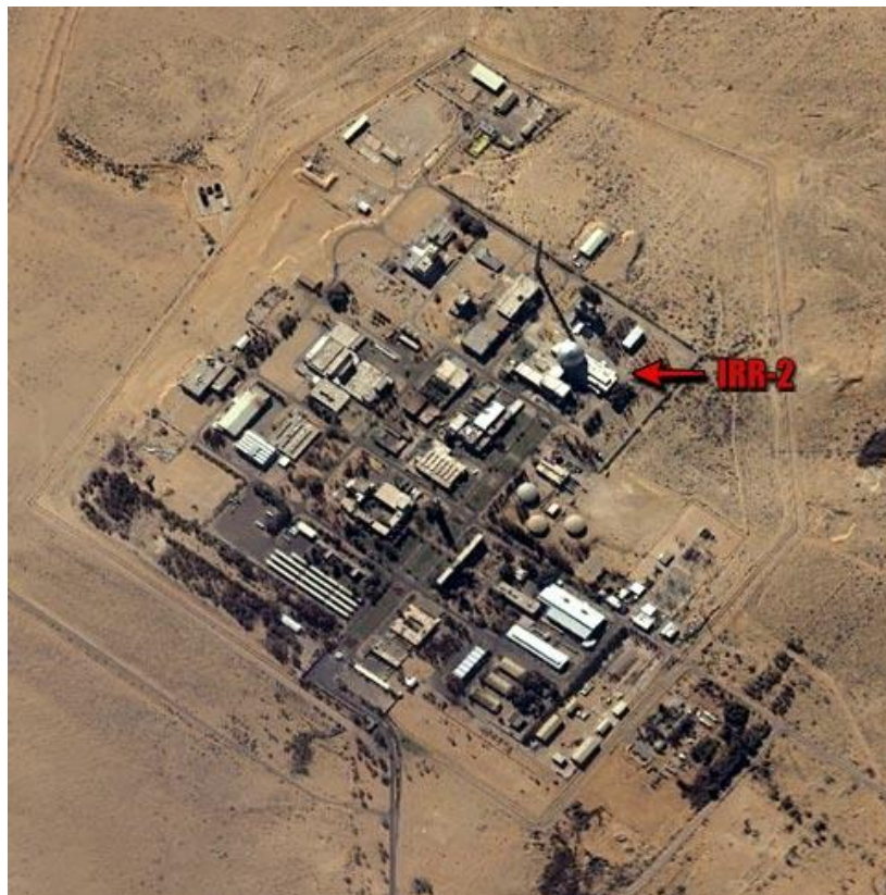
Figure 5.6 An Aerial Image of the Negev Nuclear Research Center 497
