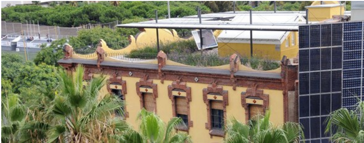
Figure 24. Image of Fabrica del Sol showing the photovoltaic and solar panels. Source: www.ajuntamentdbarcelona.cat
