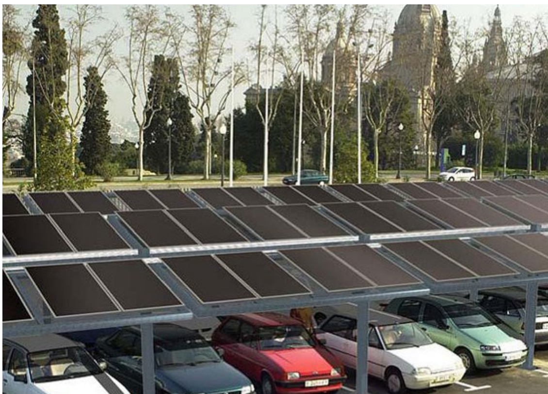
Figure 18. Solar thermal panels installed at the Olympic pool (2004). Source: Solarge Project 2008.
