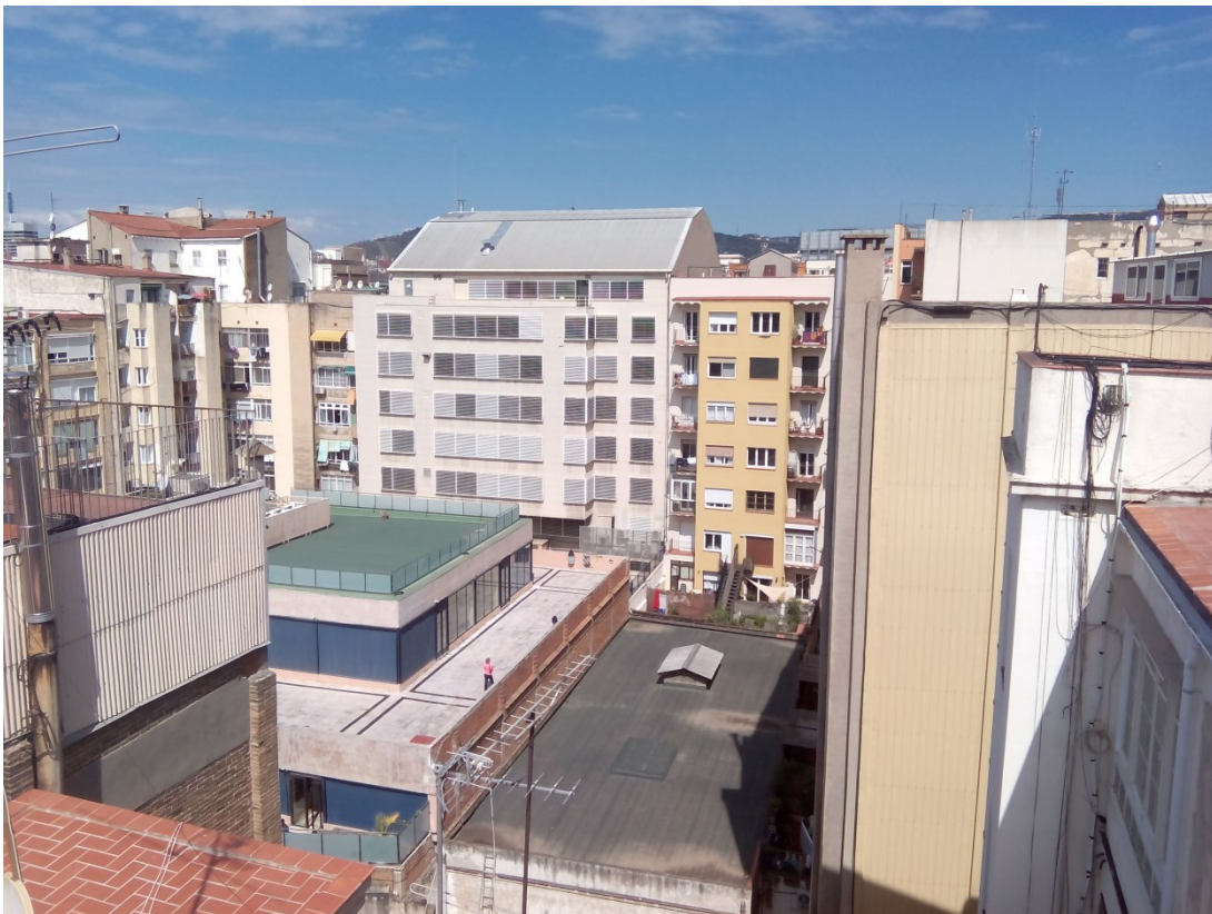
Figure 7. Interior yard of the Efficient Block .
