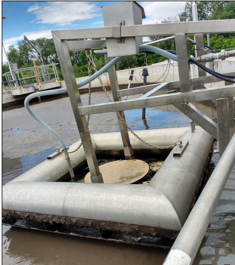
Figure 22: Biodec decanter installed in the Cyclator to decant treated water
