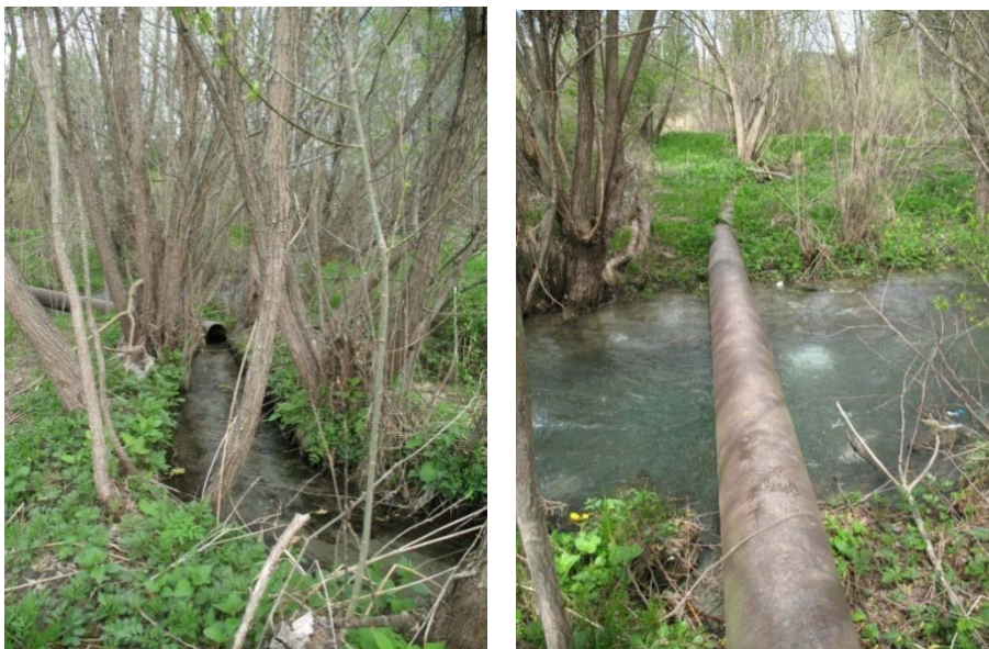
Fig. 49. The water from the canal entering the iron tube (left) water flowing through the iron tube above the mill leat towards the mill site and the abbey (right)
