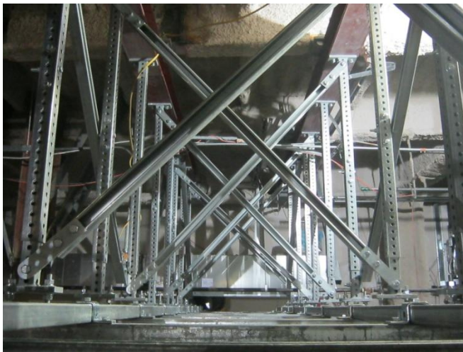
Figure 2: Cross bracing structure in construction (“Edge Construction Supply” n.d.)
