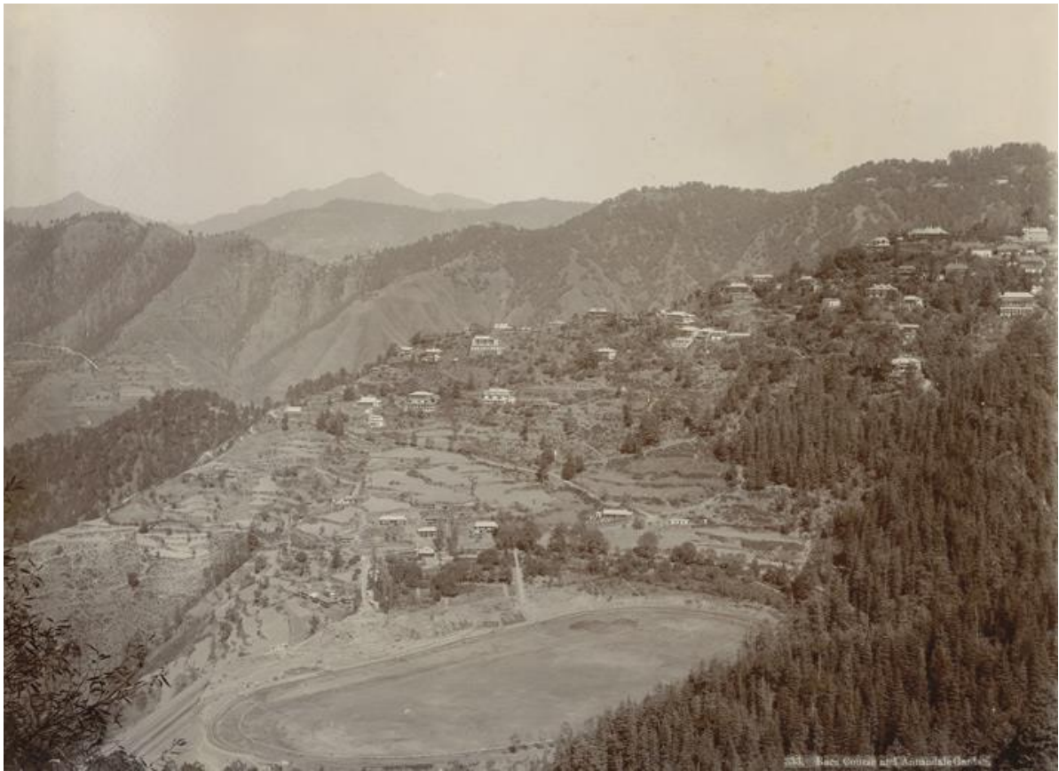
Figure 6. A view of Annadale Gymkhana from the road above, 1846. 114
