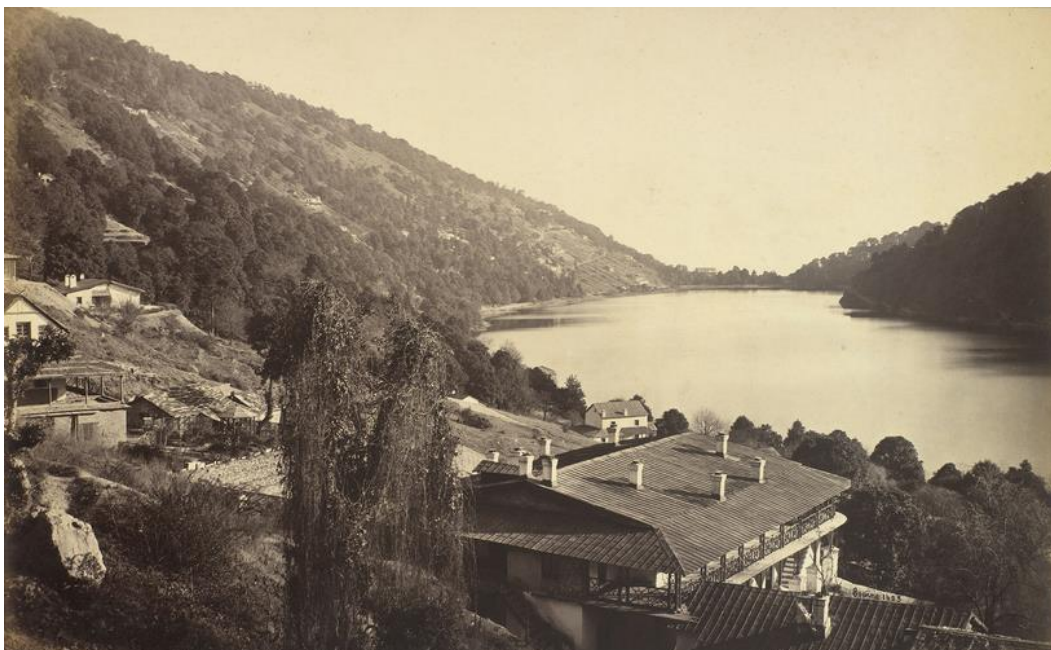
Figure 3. A view of Nainital Lake overlooking the rooftops, c.1875. 65
