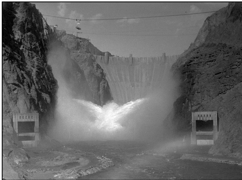
Figure 9: View showing the first time all 12 valves in the canyon wall outlets at Hoover Dam worked simultaneously, discharging Colorado River water. (1936) Courtesy of Water and Power Associates.
