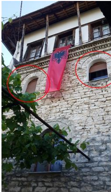
Figure 1. Salaria House, replacement of wooden windows with aluminium ones. (Photo taken by the author of the thesis)
