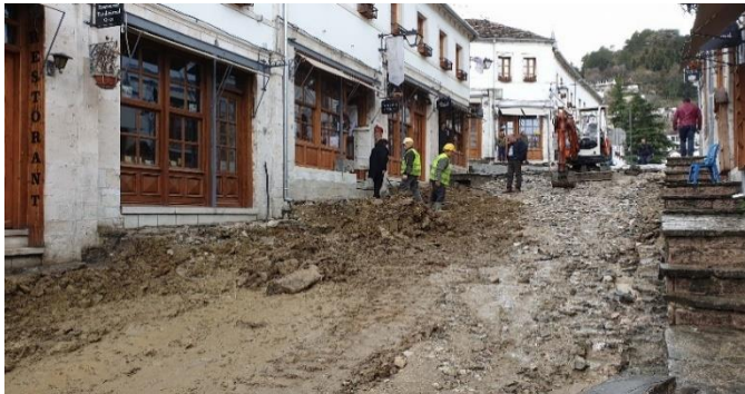
Figure 4. The process of removing the existing cobblestone
