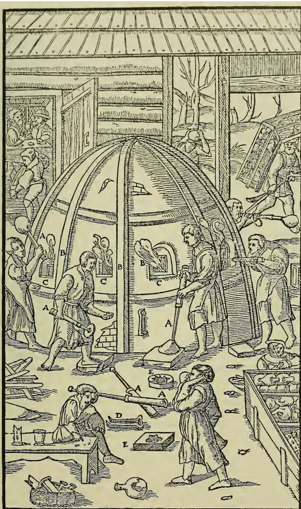
A—BLOW-PIPE. B—LITTLE WINDOW. C—MARBLE. D—FORCEPS. E—MOULDS BY MEANS OF WHICH THE SHAPES ARE PRODUCED.
