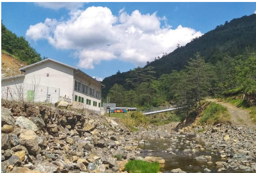
Figure 58. One of two SHPPs on the river Rzav where most of the water is directed to turbines through pipes several kilometers long, leaving the riverbed dry (Source: Marković, 2021)
