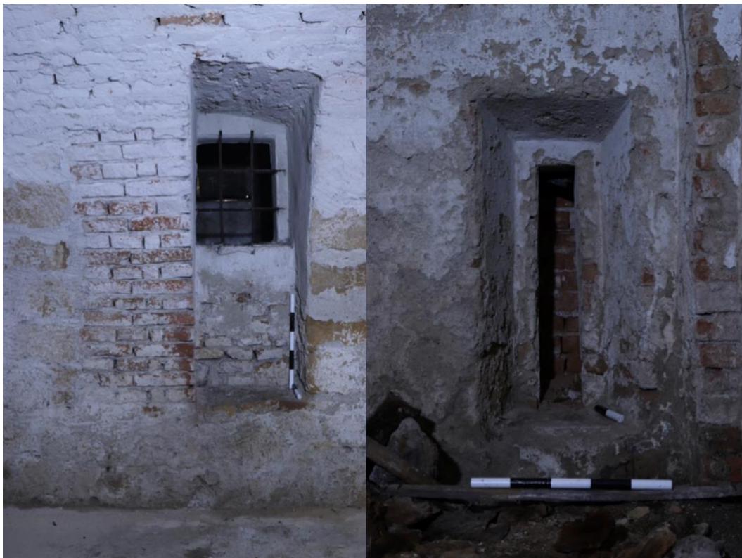
Figure 19: West facing picture of the partly bricked-up window, with its 3 stages of filling visible.
