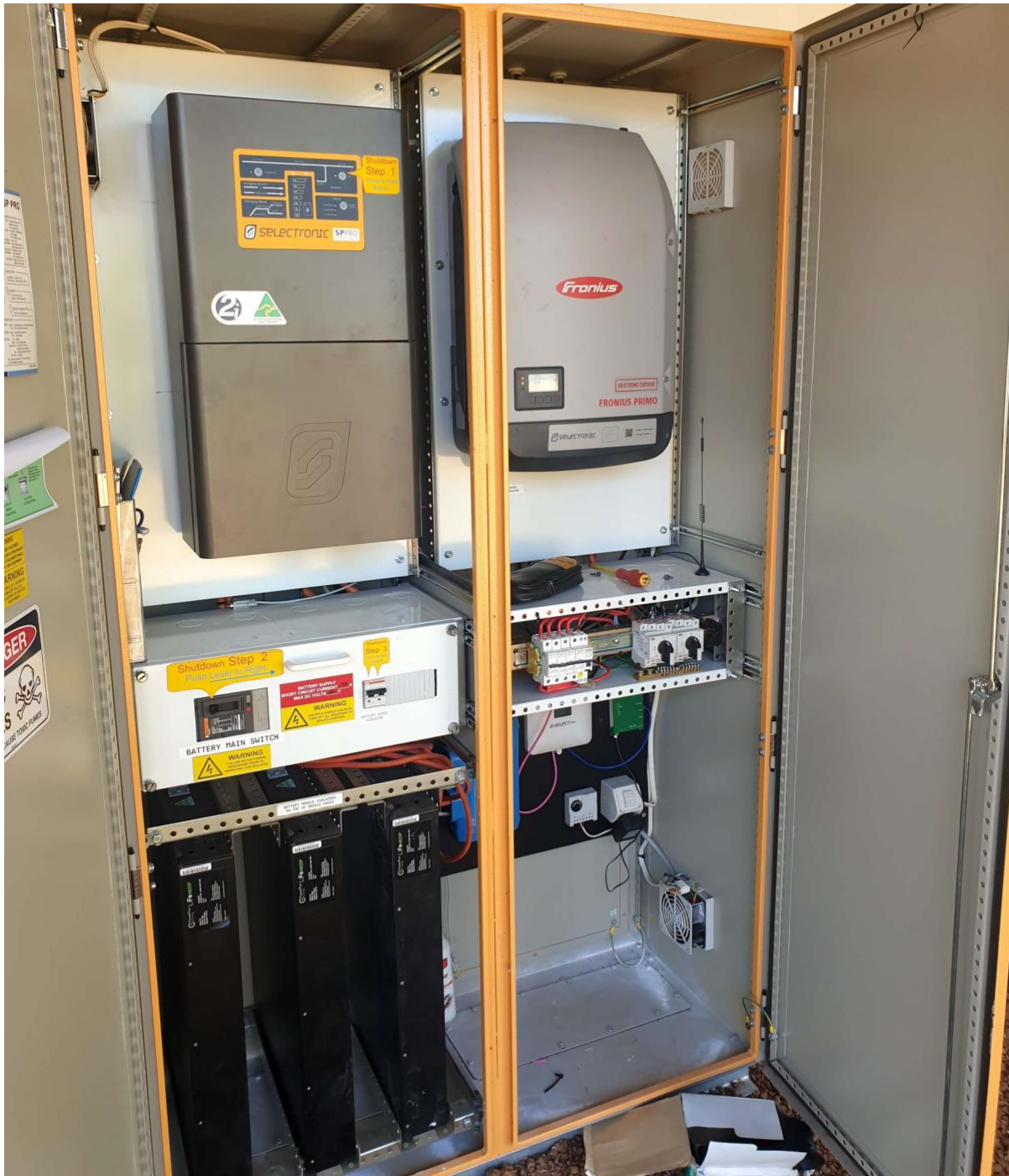
Figure 6: Battery energy storage system for Marlinja community center
