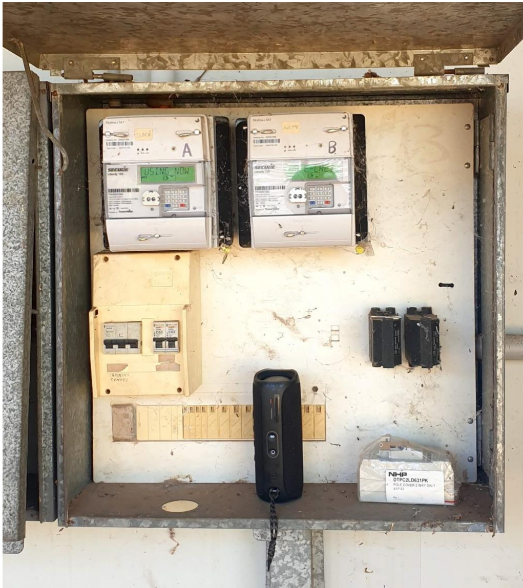
Figure 5: Prepaid electricity meter for Marlinja community center
