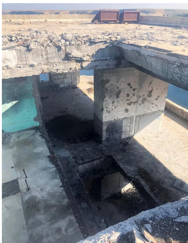
Fig. 6 A coalition missile penetrated five stories of the dam's north tower. Two missiles on the southern tower penetrated three floors down Source: Azmat Khan, The New York Times
