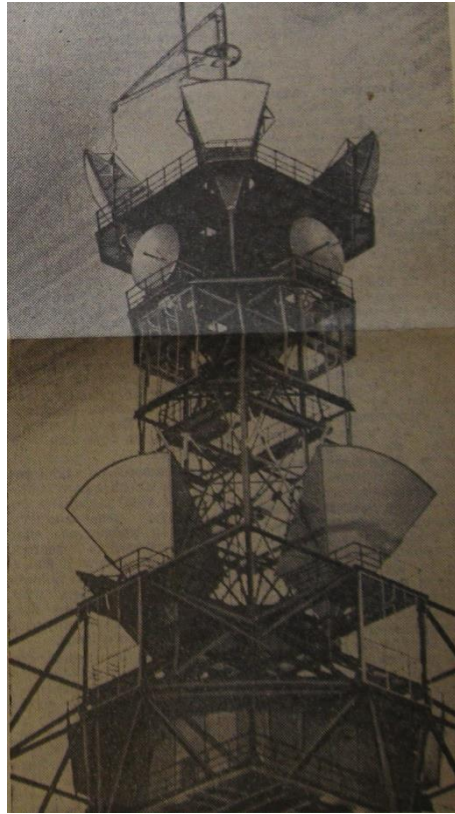
Figure. 2.3. An experimental multi-channel communication station designed for radio, television, telegraph, telephone and phototelegraph. Sovetskaia Rossia 6 May 1968 in: HU OSA 300 - 80 – 1, box. 765
