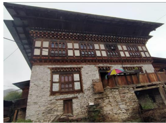
Figure 14. House with fewer openings and more walls on lower levels, and fewer walls and more openings on upper levels (Picture by author)
