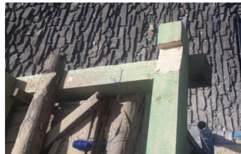
Figure 14: Replacement of the wooden beam, Image taken by the writer of the thesis.
