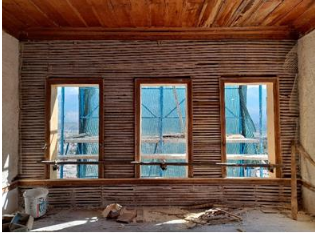
Figure 13: Restoration of çatma and preparation of plaster for çatma, 2022.
