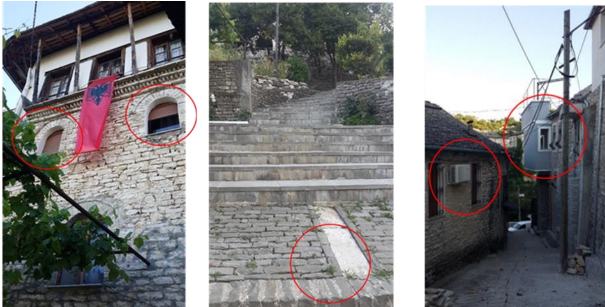
Figure 22: The illegal interventions in the historical buildings, first category monuments of culture, and alleys (different materials from the original – aluminum windows, white tiles instead of white cobblestone, additions of the existing building with new materials, and changing the façade of the building), district “Partizani”, Gjirokastra.
