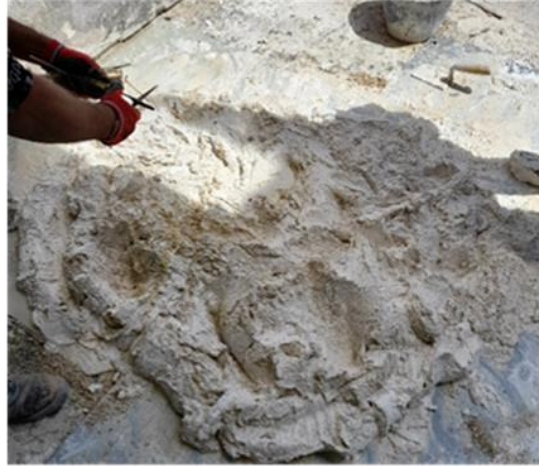
Figure 13: Restoration of çatma and preparation of plaster for çatma, 2022.
