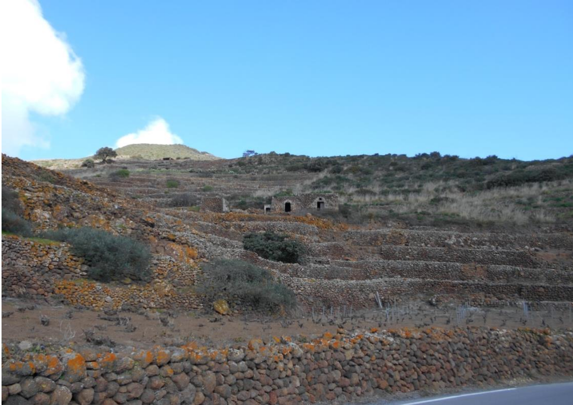
Figure 17: Dry-stone wall system. It can be seen in this image that the dry-stone wall system is not only an infrastructure but also an integrated system that contributes to the creation of an organic landscape (Photo by the author, 2024)
