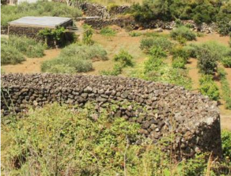
Figure 18: Sloped top edge detail. This photograph clearly illustrates what is meant by an inwardly sloping edge that can dampen wind effects and protect the plants inside the garden (Photo courtesy of Legambiente)
