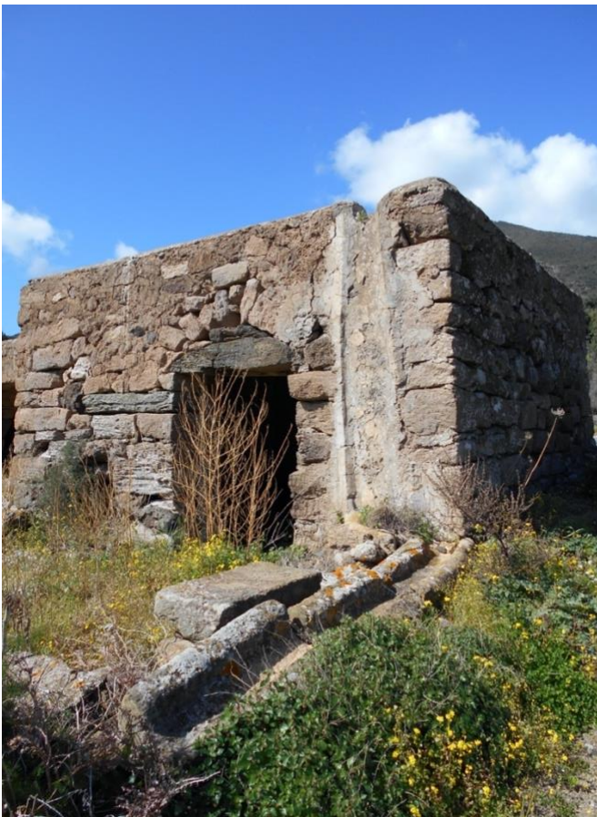
Figure 31: Kannalláte. It is possible to see here the channel that brings the water down, and it is the same in many cases. It was also intended to water the animals, otherwise, it would not be open (Photo by the author, 2024)
