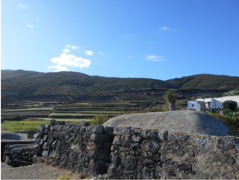
Figure 28: Vaulted roof. Every dammuso or small building has a vaulted roof, there are very few exceptions, any such roof implies water collection (Photo by the author, 2024)
