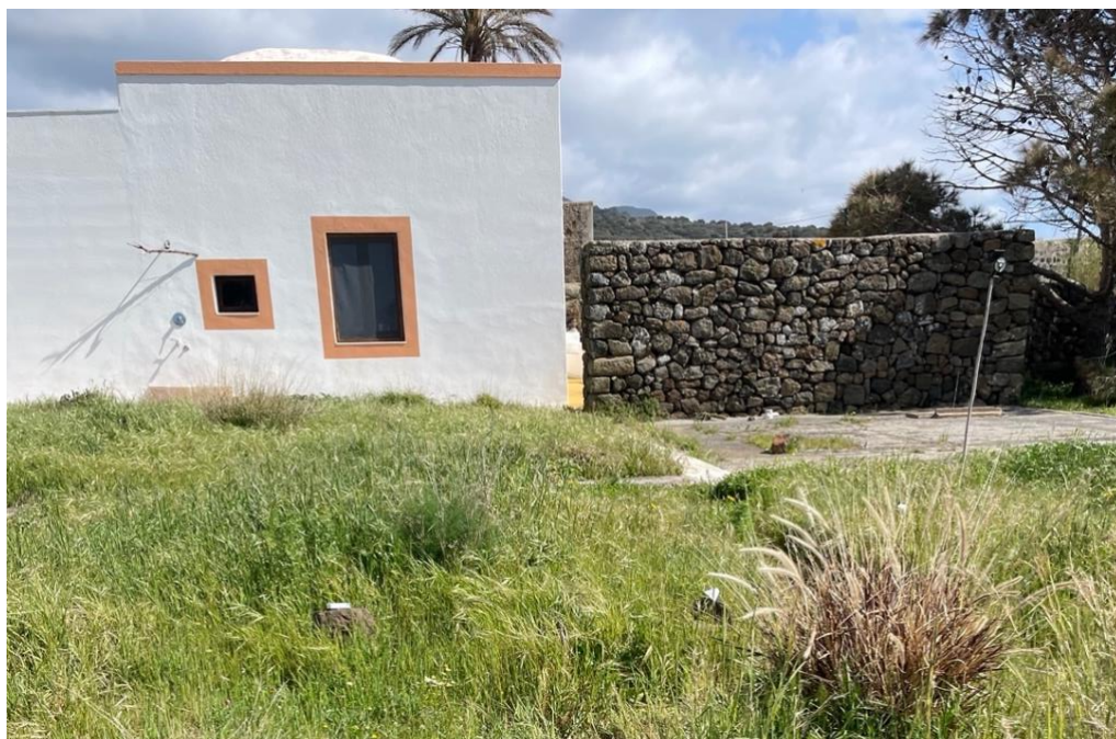
Figure 26: Cistern. At the bottom right, you can see the cistern; the one on the left was my dammuso, and the one on the right is a dry-stone wall. Again, you can see that everything is close together and connected and valuable for water collection (Photo by the author, 2024)
