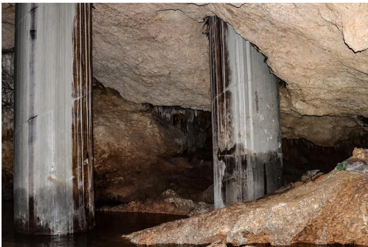
Figure 6 Cement pillars drilled into a cave.
