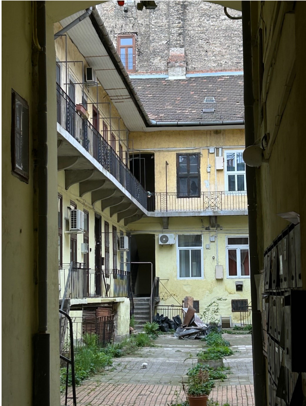
16. Figure: Passing in front of apartments on the circular corridors, one might notice the mosaic-like installation of outdoor units belonging to entirely different heating devices: a condenser for an air conditioner mounted on the wall of one apartment and a cone-shaped metal structure that forms the outer end of a flue for a type of gas-fired central heating appliance, on another. (Photo by author).
