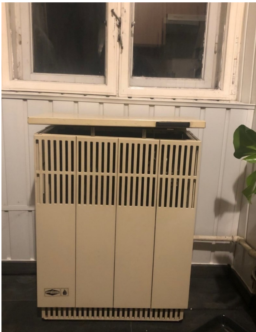
18. Figure: The heating device in Boró and Lilla's kitchen. A gas fitter recommended that it should be never kept off, because there is a chance it might not turn on again the next time. It had been running throughout the entire heating season, and never did it come close to being even lukewarm to the touch. (Photo by author).
