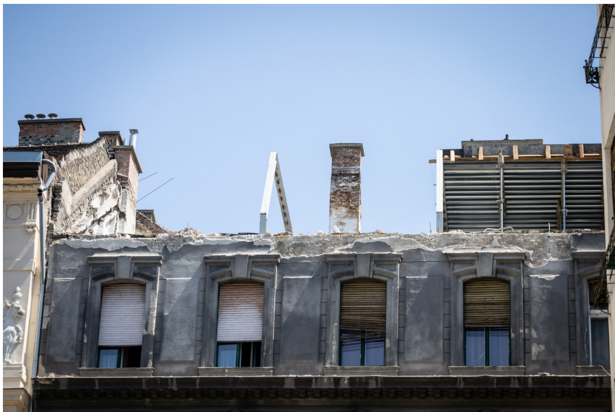
1. Figure: Close-up of the remains of the collapsed roof structure of the Jókai Street residential building. (Photo by Zsófi Szollár / Index.hu)
