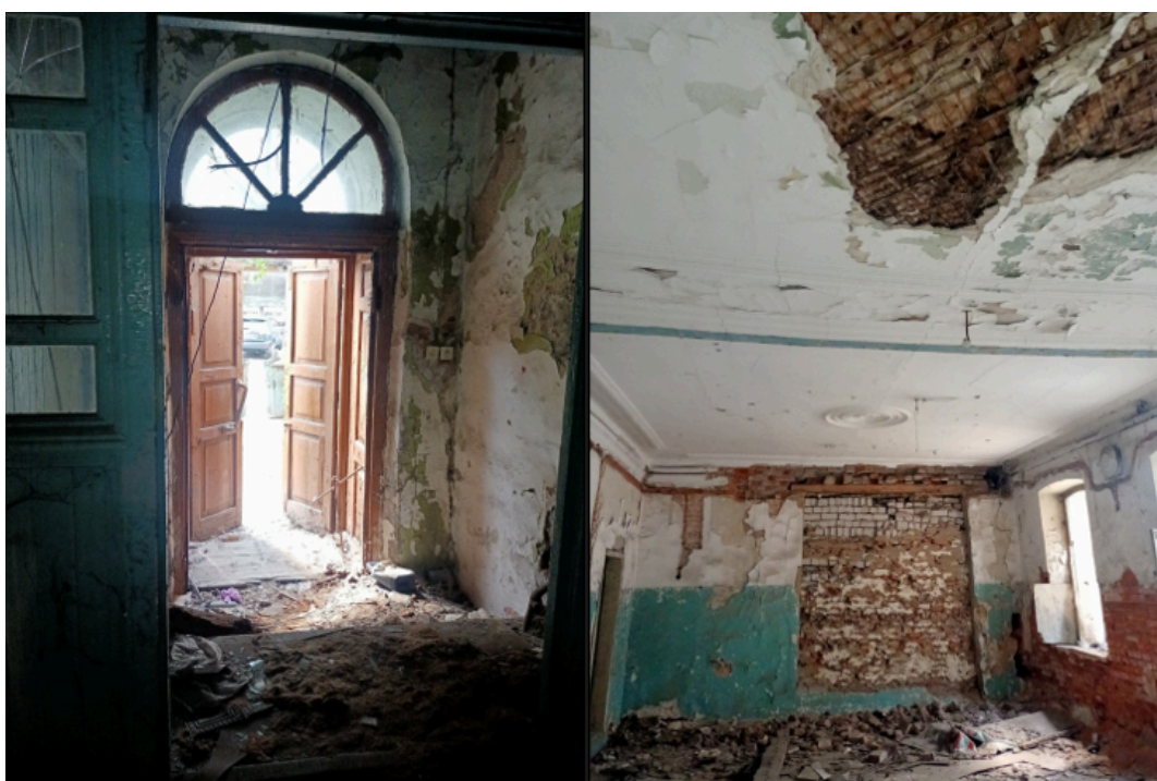
Figure 4. Interior of the Central Telegraph Building.
