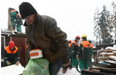
Figure 16. “ Vilniaus tabore griaujami neteisėti statiniai ” [Illegal Structures Are Being Demolished in Vilnius Camp], Delfi , February 13, 2012, accessed May 9, 2025, https://www.delfi.lt/news/daily/lithuania/vilniaus-tabore-griaujami-neteisėti-statiniai-55424885 .
