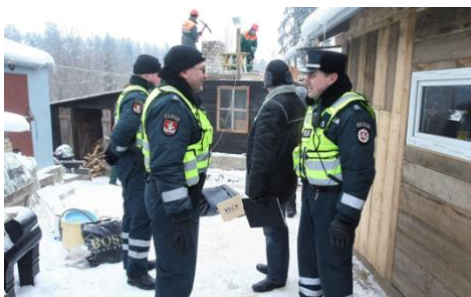
Figure 15. “ Vilniaus tabore griaujami neteisėti statiniai ” [Illegal Structures Are Being Demolished in Vilnius Camp], Delfi , February 13, 2012, accessed May 9, 2025, https://www.delfi.lt/news/daily/lithuania/vilniaus-tabore-griaujami-neteisėti-statiniai-55424885 .
