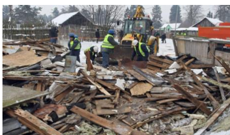
Figure 17. “ Vilniaus tabore griaujami neteisėti statiniai ” [Illegal Structures Are Being Demolished in Vilnius Camp], Delfi , February 13, 2012, accessed May 9, 2025, https://www.delfi.lt/news/daily/lithuania/vilniaus-tabore-griaujami-neteisėti-statiniai-55424885 .
