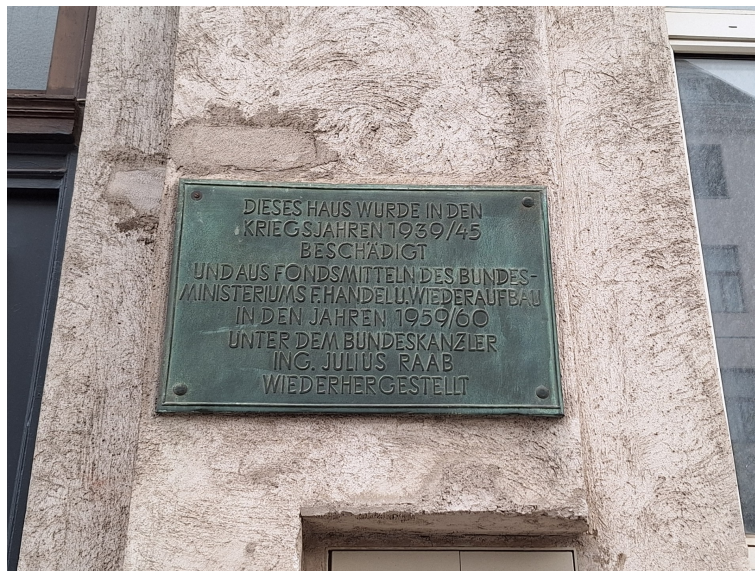
Figure C.5: Plaque on a rebuilt housing estate
