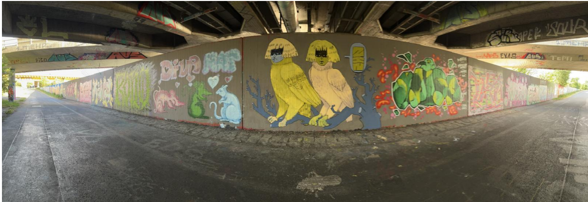
Figure 3. At the Hall of Fame at Nordbrucke, these walls are in much better condition than the more used walls along the Donaukanal (photo by author)
