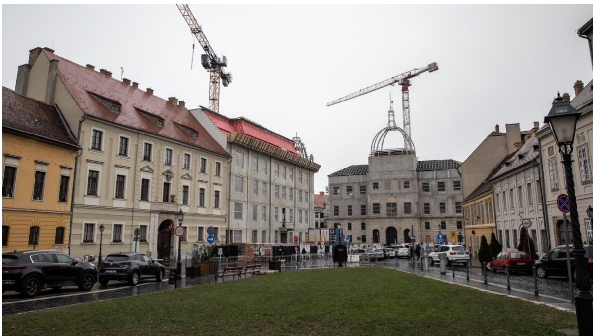
Figure 23. The Construction of the former Ministry of Defense in 2023. valaszonline.hu
